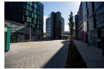
Abbildung 4 Bainfield Student Accommodation
