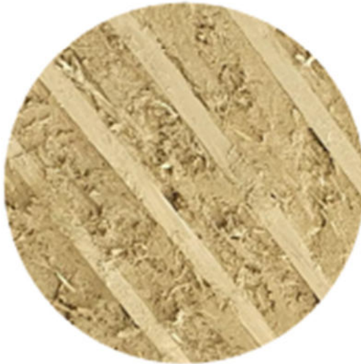
First layer plaster
