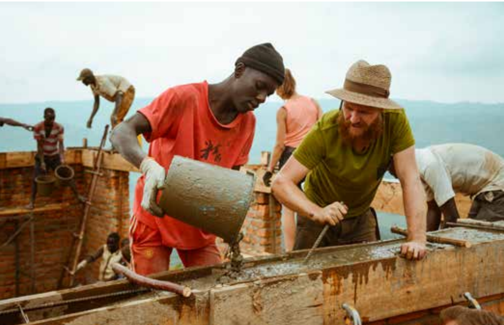
Ringanker betonieren Concreting the ring beam
