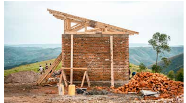
Konstruktion: Fundament, Ziegelmauer, Beton-Ringanker, Dachbinder Construction: foundation, brick wall, concrete ring beam, roof trusses
