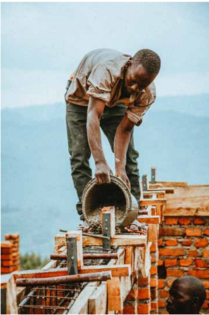
Ringanker betonieren Concreting the ring beam
